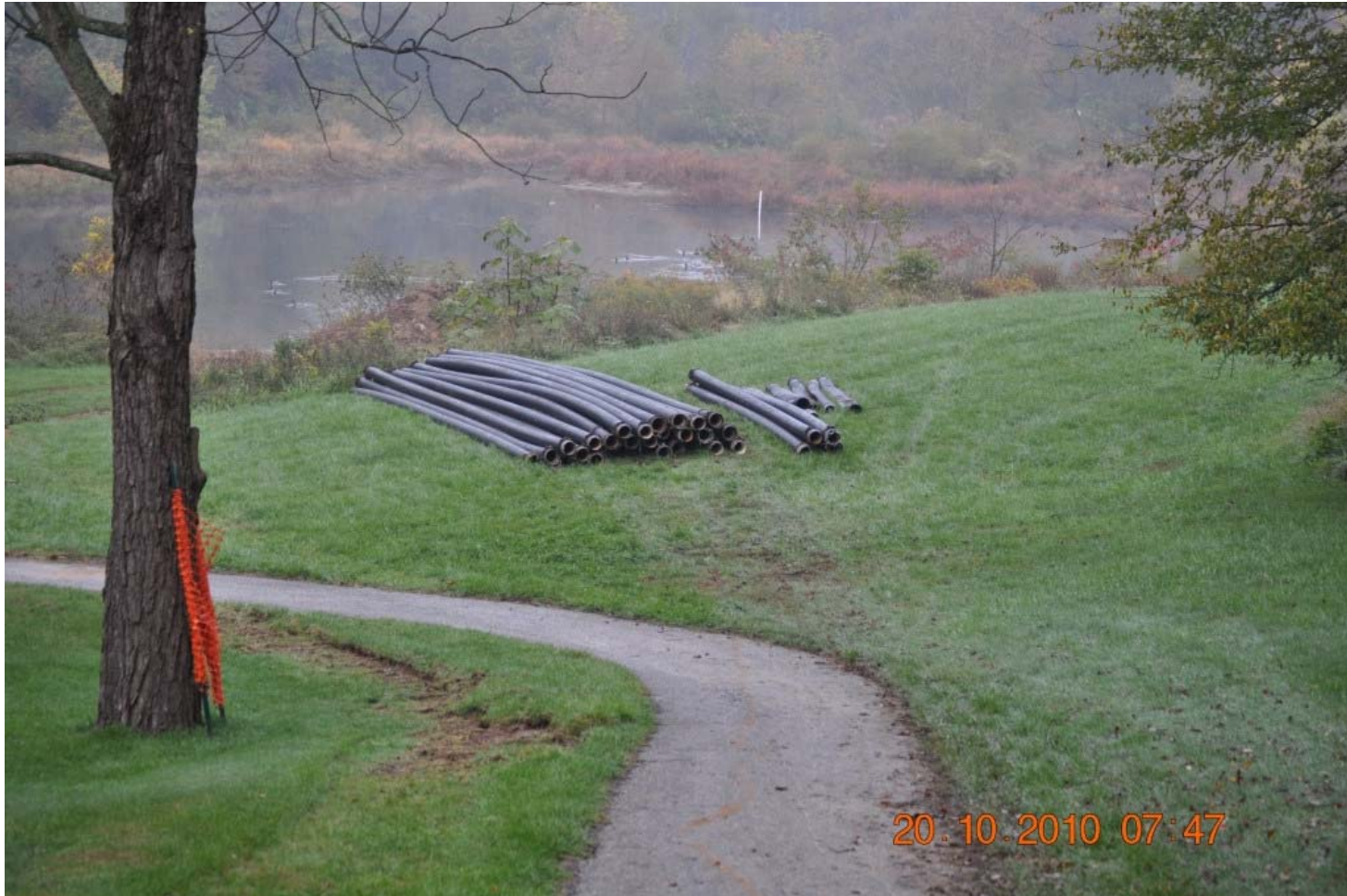
October 20 – Area 1 piping
