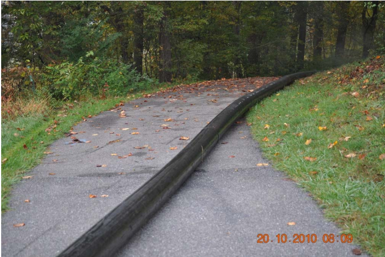
October 20 – Dredge piping Area 1 to Area 2
