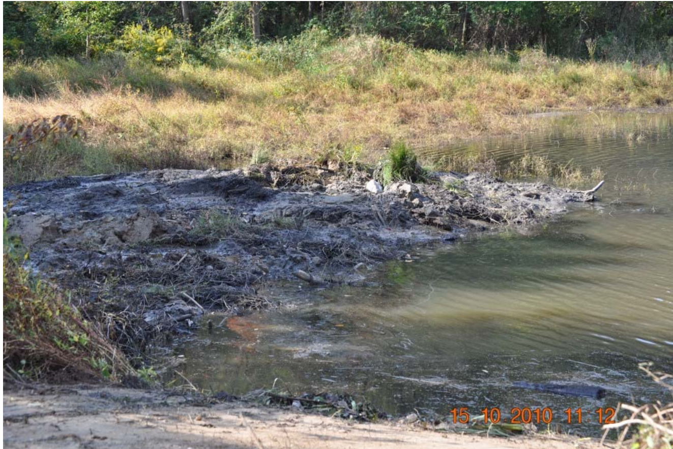
October 15 – Area 1 excavation for dredge placement
