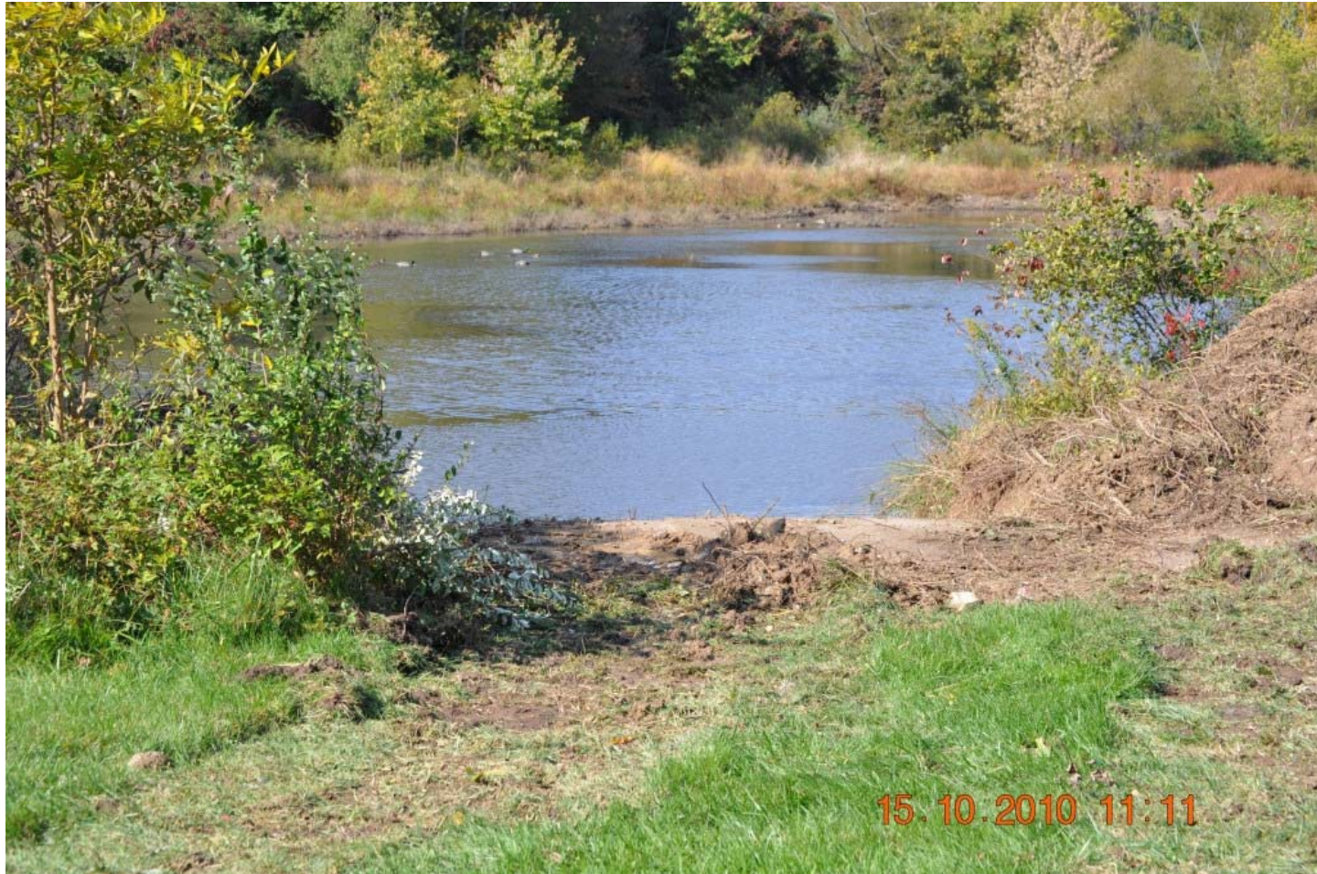
October 15 – Area 1 Forebay Pond
